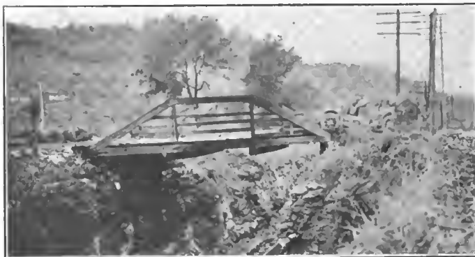
Crossing a Viaduct Nine Miles out of Franklin, Tenn.
